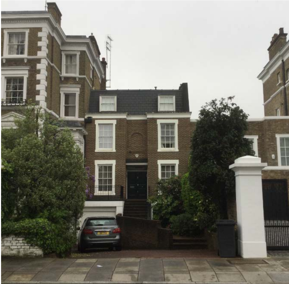
Front of Application Site
